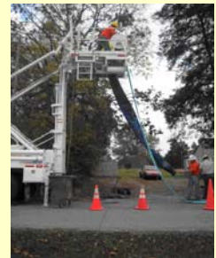
Installation of competing CIPP liner
