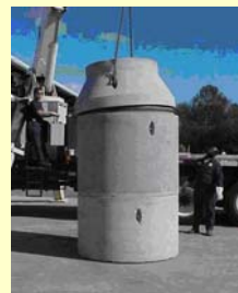
Installation of a new precast concrete manhole
